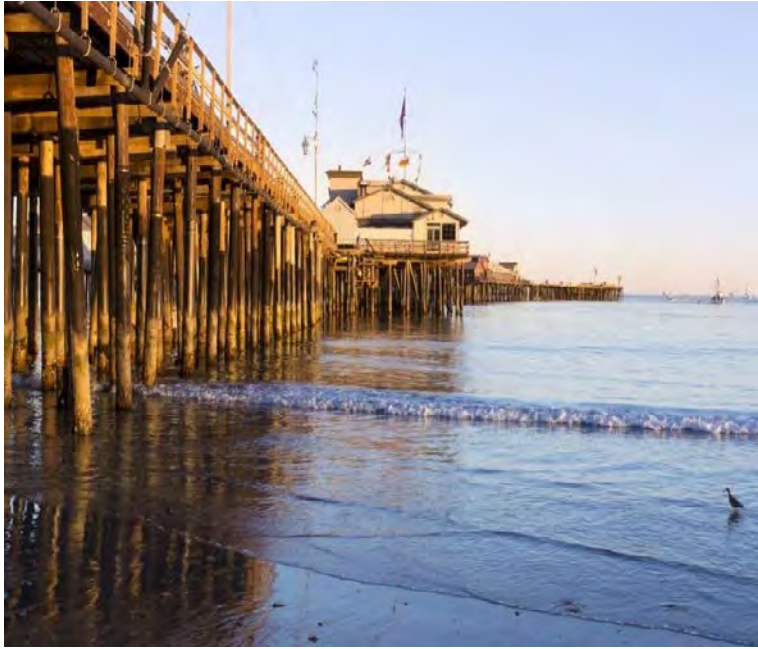
Santa Barbara Stearns Wharf
